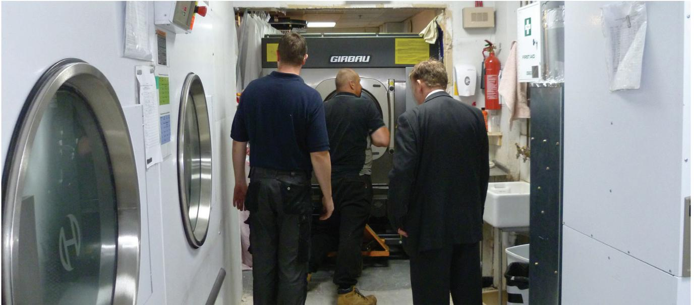
The laundry operates every day of the year and Girbau was able to install the new machine in just a 5-hour window at the weekend, in order to keep disruption to a minimum. A delivery truck with HIAB crane was used to lift and then lower the washer carefully through a basement window. A section of firewall had to be temporarily removed and replaced as the washer was carefully manoeuvred into place, before being connected to services and commissioned.
