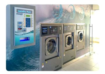
The laundry is equipped with two HS-6008 (9kg capacity) washers, a HS-6013 (14 kg capacity) washer and a HS-6017 (19 kg capacity) washer. It also has two ED260 (13kg capacity) dryers and a central payment unit.
